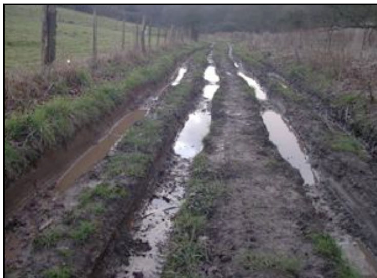
Wiltshire Byway, severely damaged by off-road motor vehicles, before reinstatement.
